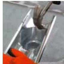
Next connect the 2 inner marks by drawing a circle between them (Fig.4). Make an initial hole with a drill or hacksaw and then with a pair of good quality tin snips cut the circle out that you have marked (Fig.5) re-attach outlet; fold rear tabs of outlet over rear edge of gutter and tap the inner rough edges of cut whole into the outlet with a hammer (Fig.6)
