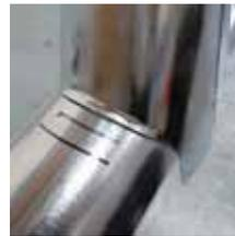
First insert the front lip of the wrap around outlet into the front roll of your gutter in the desired position along its length (Fig.1) mark a line either side of your outlet (Fig.2); then move the outlet inward by 20mm and draw a further line leaving 2 clear marks (Fig.3)
