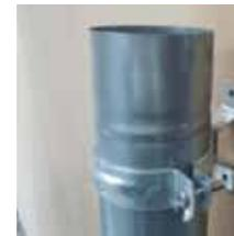
Offsets are achieved using 2No 70° bends (Fig.8) with larger offsets being made by inserting a length of pipe in between the 2 bends; Downpipes are fixed/held by 2No downpipe clips (Fig.9)
