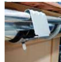
Insert bead connector into front roll of gutter & locate next section of gutter or gutter fitting onto bead connector (Fig.4) locate gutter connector over rear edge of gutter allowing for expansion gap indicated by notch cut in rear of union (Fig.5) push down on top clip at front of connector and squeeze clip shut. Fold locking tab over to fully secure (Fig.6 & Fig.7)
