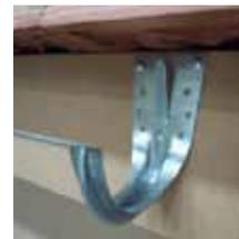
Using a plumbline mark out the position for your fascia brackets along the run. Install fascia brackets using 5No SCREW15; 2 screws should be used on both the left and right fixing options and 1No screw in the lower fixing hole underneath the gutter securing tab (Fig.7 & Fig.8)
